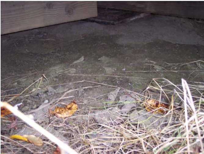
Photograph 3 – Ground Surface Beneath Fuel Tank
